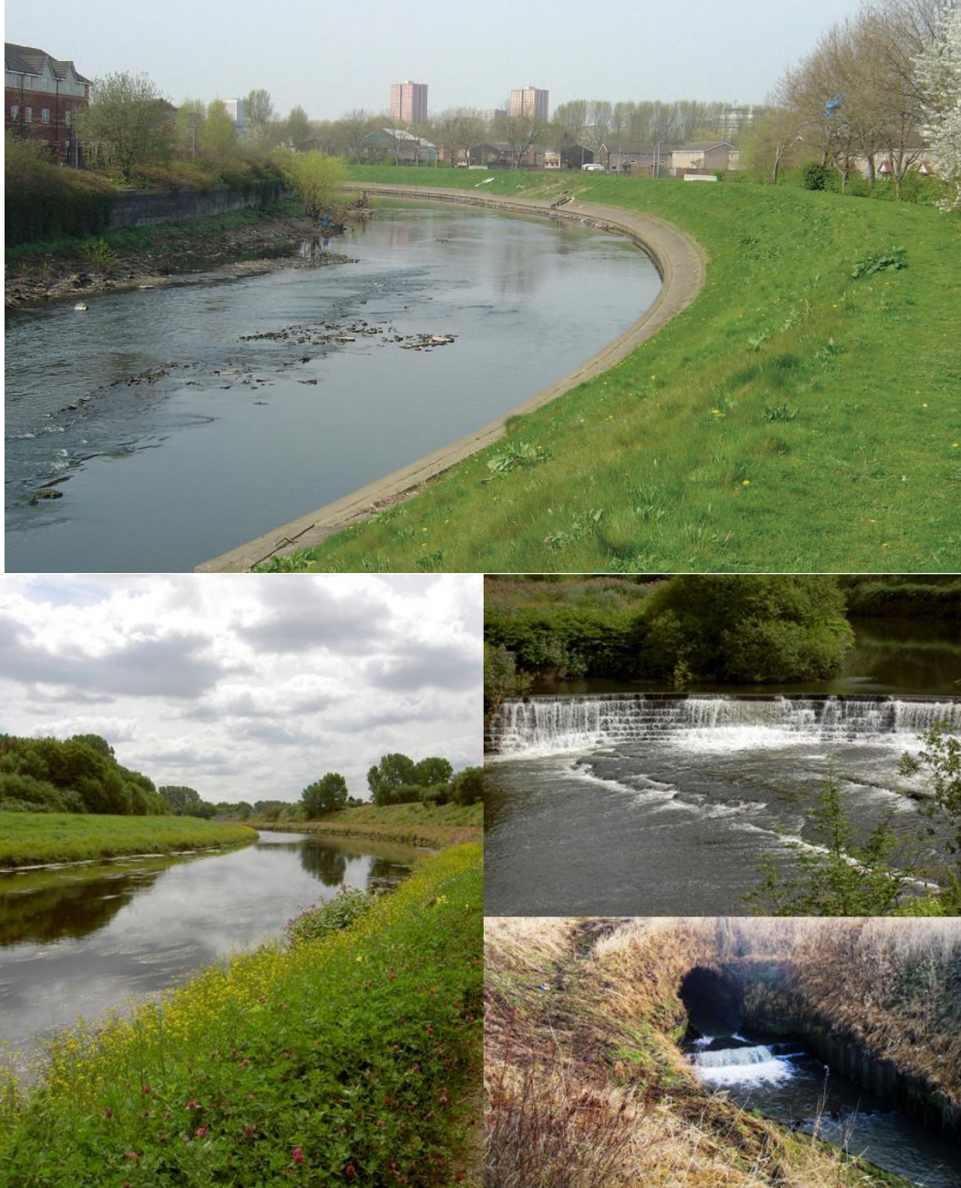
Figure 9 Examples of physical modification (top and left – flood embankments, middle right - weir, bottom right – culvert) 17
