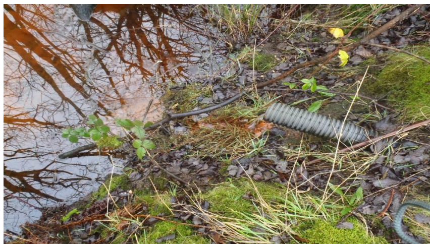
Figure 25 Land drain on old landfill site discharging into Middle Brook 40
