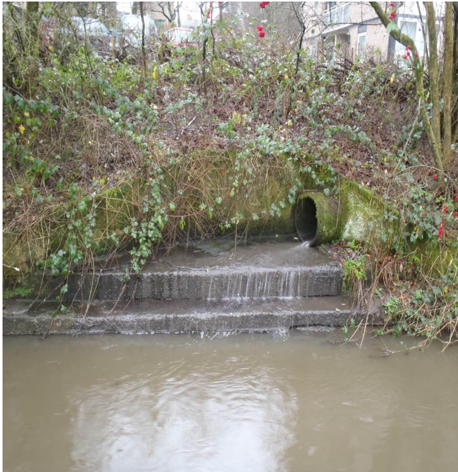
Figure 20 Surface water drain with sewage discharge probably from wrongly connected foul waste pipe 34
